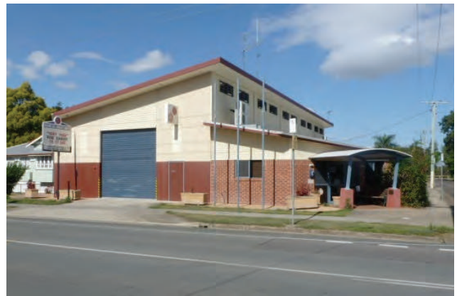
Emergency Services Building 2012
