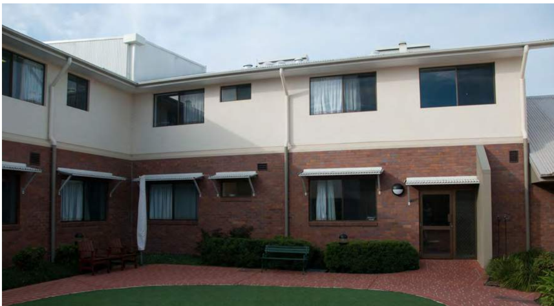
Viewing the high care wing from the courtyard.
